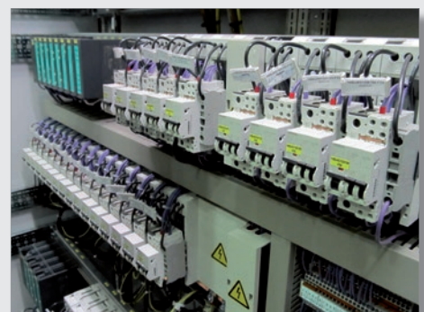
Image 8: Direct current distribution
