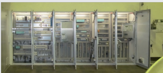
Image 9: Central control system hydropower plant Schwammenauel
